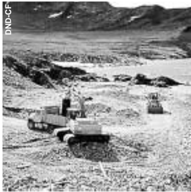
Clean-up site in Saglek, Labrador.
